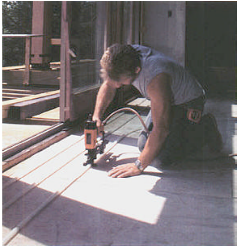
Radiant floors can be installed almost anywhere. Radiant tubing is pneumatically stapled to a conventionally framed plywood subfloor before being covered with a thin concrete slab. Flooring choices include wood or carpet.
