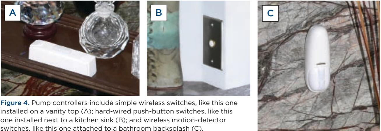
**Figure 4.** Pump controllers include simple wireless switches, like this one installed on a vanity top (A); hard-wired push-button switches, like this one installed next to a kitchen sink (B); and wireless motion-detector switches, like this one attached to a bathroom backsplash (C).
