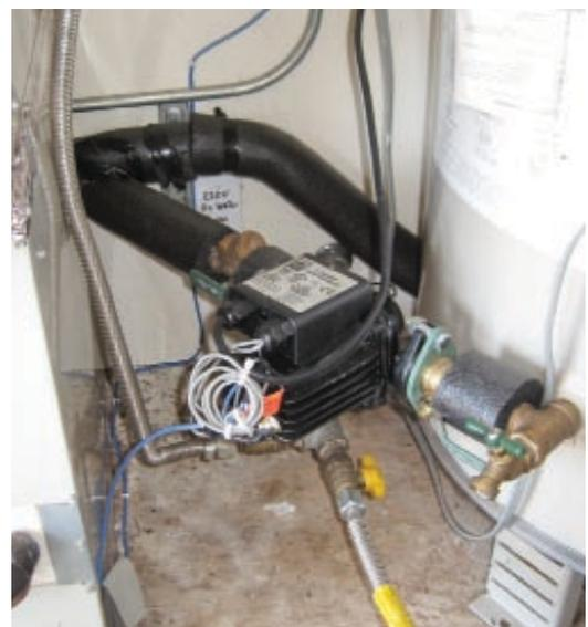
**Figure 3.** When possible, the author prefers to install the on-demand circulating pump at the water heater in a closed-loop configuration. The pump can be activated by any number of manual switches or motion detectors located near fixtures on the hot-water line.
