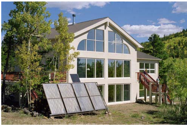
Figure 2. View of home from the southwest, showing the significant south-facing glazing for passive solar heating and the solar hot water collectors in the foreground. The 1,000-watt photovoltaic array east of the house is not shown in this view. (NREL PIX 08226)
