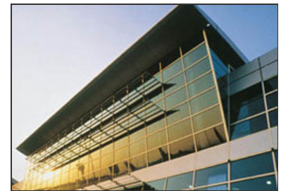
International terminal building in Istanbul's Ataturk Airport uses laminated glass for safety and security (Courtesy of DuPont Laminated Technologies)
