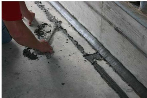
Figure 17: Grouting of anode and lead wires in ECM floor.
