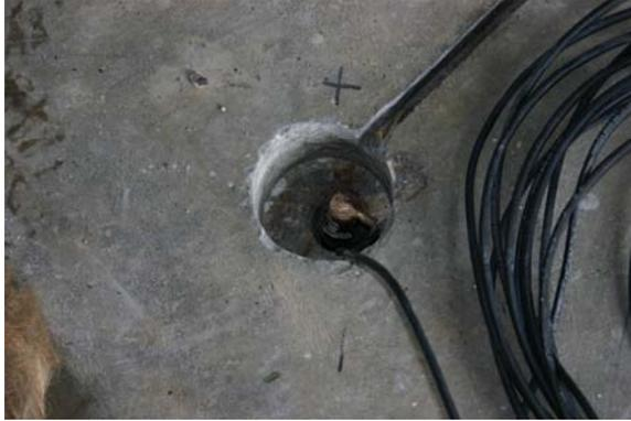
Figure 16: Cathode placement through the floor to the exterior of the ECM
