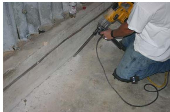
Figure 15: Chipping of 1/2-inch deep groove for anode placement.
