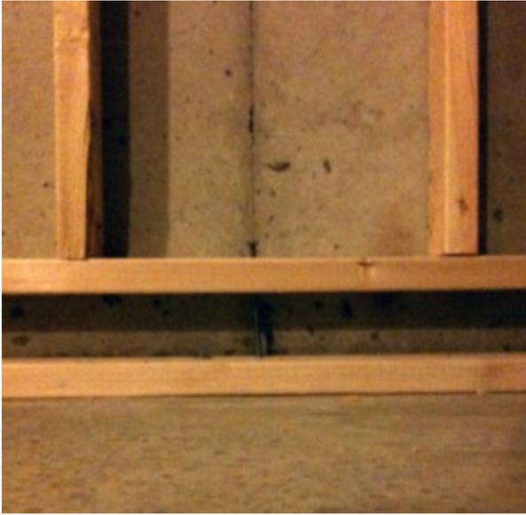
You now have a floating wall (you can also think of it as a hanging wall). As you will see, nothing is attached to the bottom base plate except the 60d nail. The nail will act as a guide rod should the concrete basement floor start to rise. However, it will not lift the top base plate because the 2x4 studs running to the ceiling are holding the top base plate in place.
