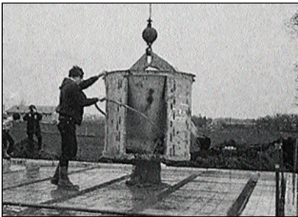
Figure 3. Because of muddy site conditions concrete was placed with a crane and bucket.
