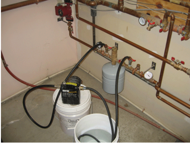
A 1/2 hp utility pump is ideal for filling a closed system.
