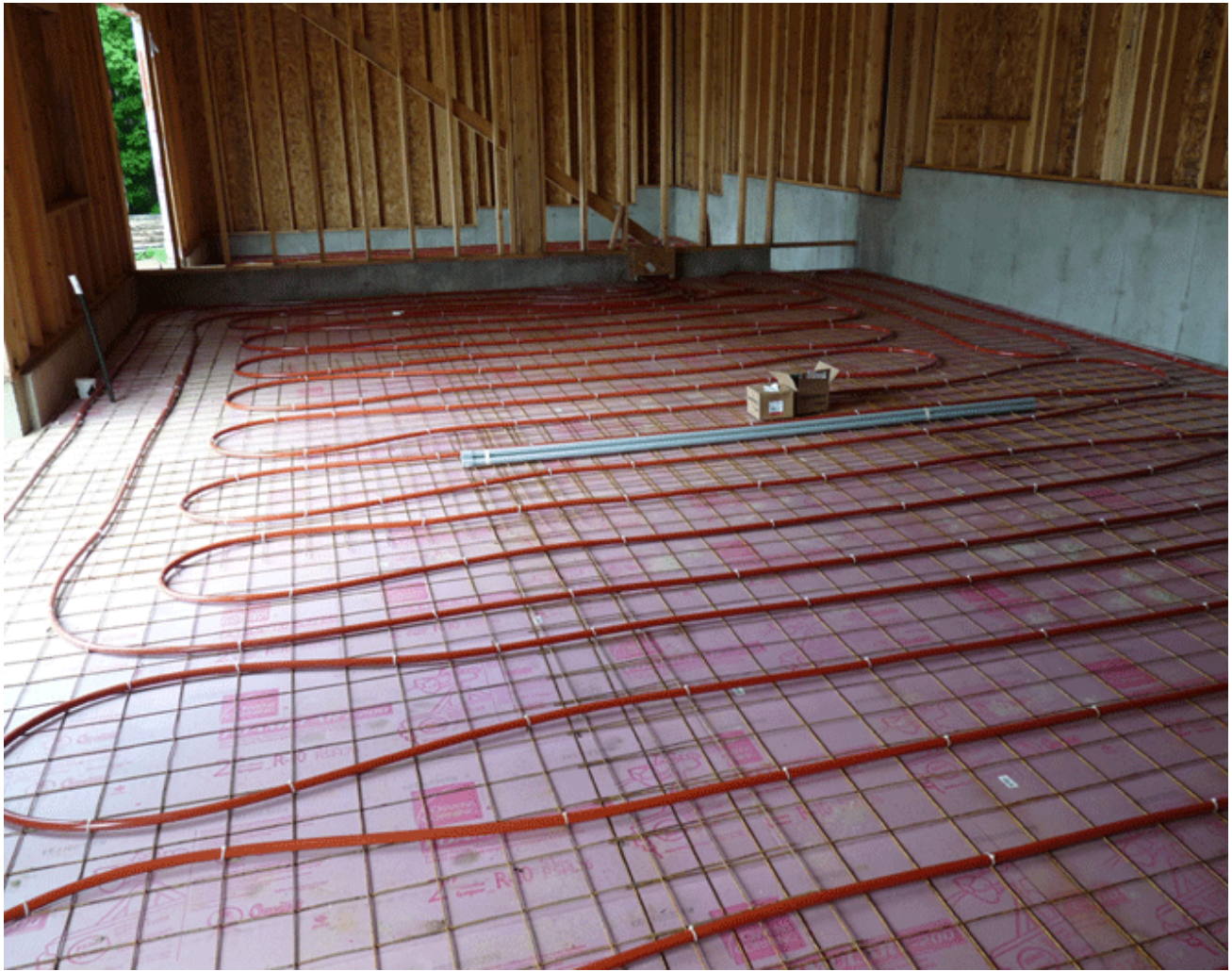
Future workshop slab prepped with insulation, wire mesh, and 7/8" Durapoly XL PEX.
