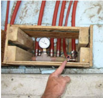
The "sensor sleeve" installed in the manifold box
