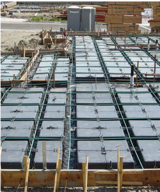
Figure 1 | Wafflemat foundation forms, ready for concrete pouring. Post-tensioning cables are positioned in the spaces between the Waffleboxes.
