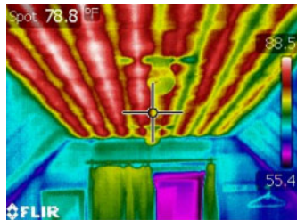
thermal image of ceiling in operation
