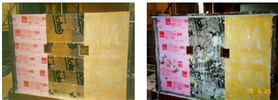
Before Installing Brick
