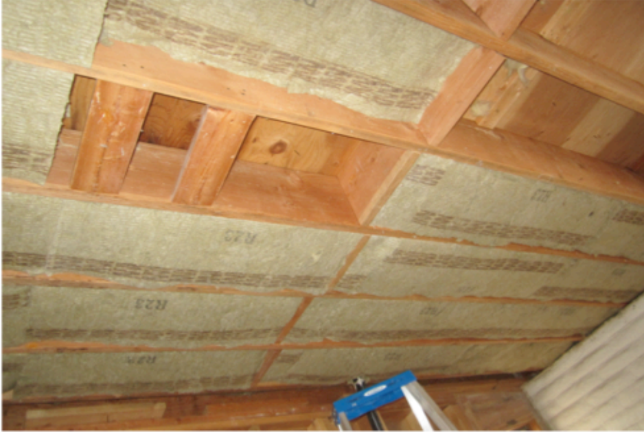
New Roxul rock wool insulation is installed in ceilings and walls.
