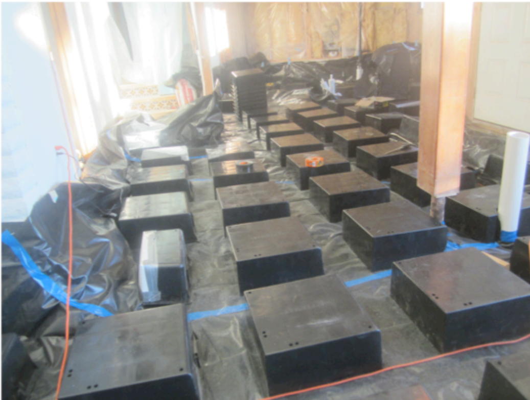
Recycled plastic "waffle boxes" were installed over a machine tamped gravel bed and a 10 mil plastic vapor barrier that was overlapped and taped at the seams and around all plumbing penetrations.
