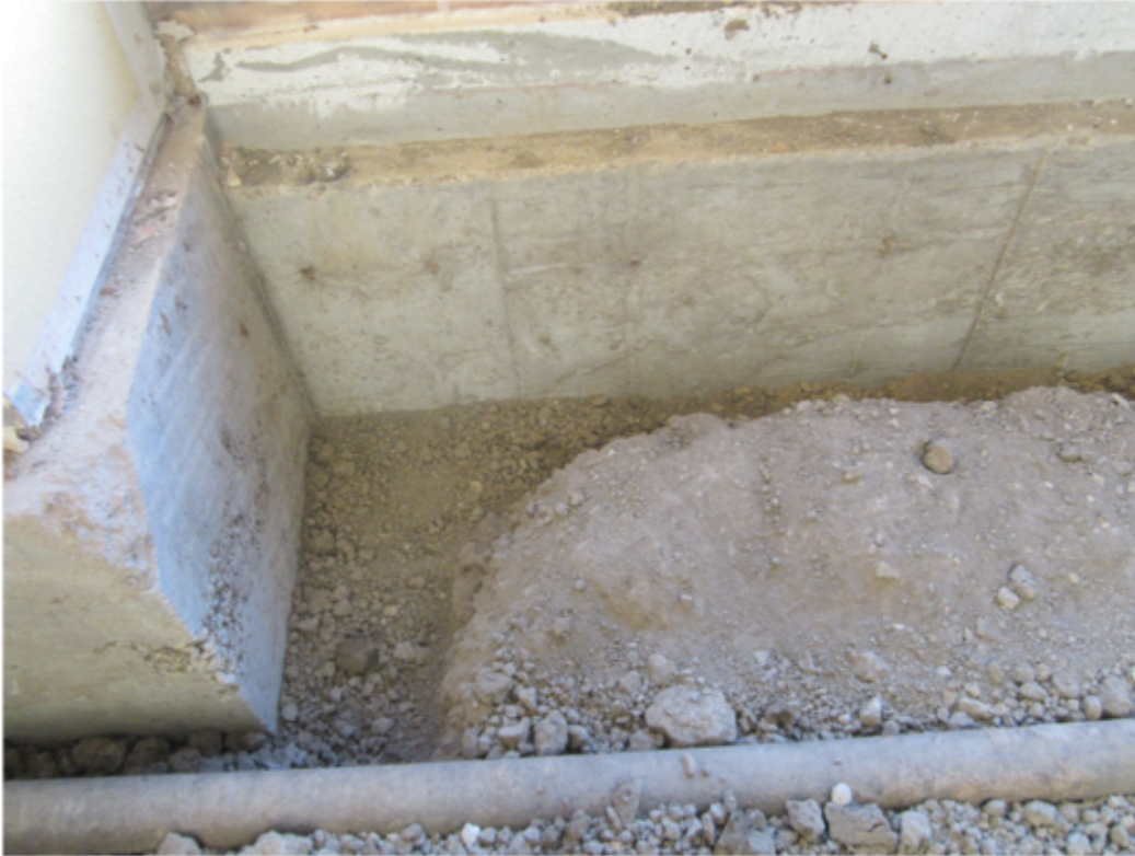
Interior foundation walls were excavated 24" to install XPS insulation board.
