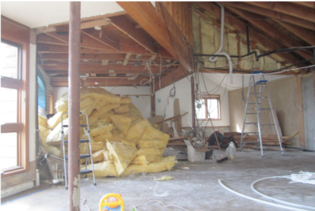
Fiberglass batts and plastic removed from slab area ceilings. The best batts were saved to provide more insulation for the remaining attic area.
