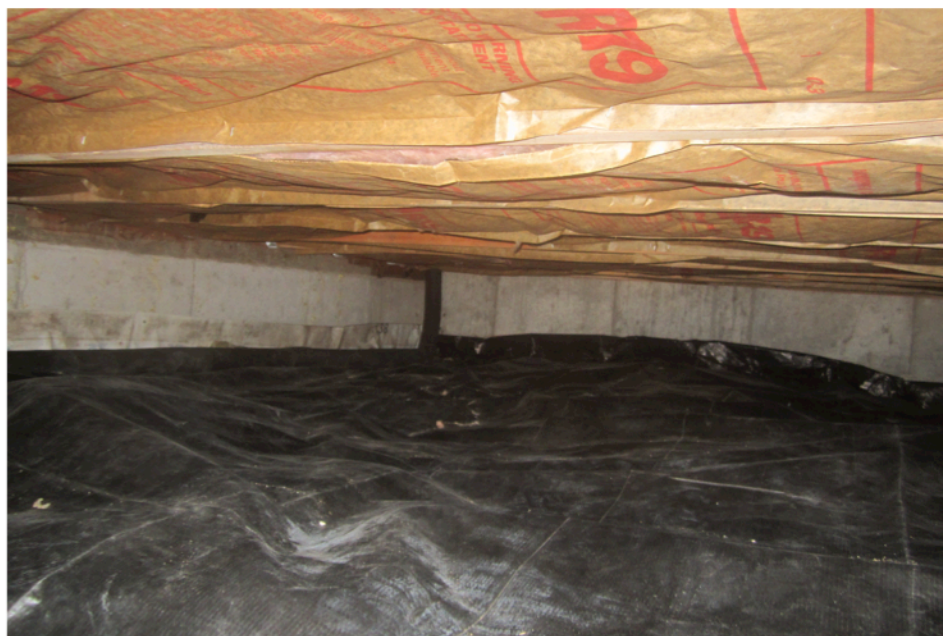
Heavy vinyl vapor barrier installed in crawlspace.
