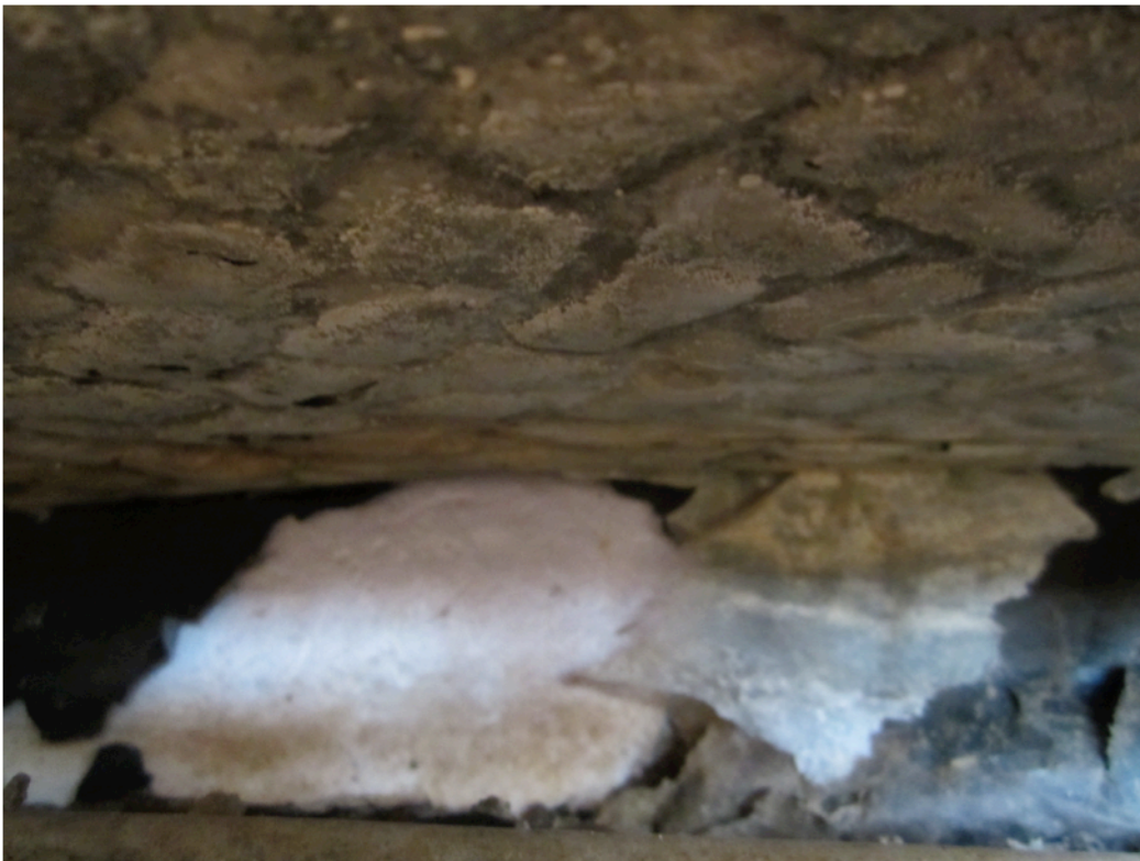
The space under the poured concrete walls between the cassettes in the foundation was dug out and revealed the polystyrene insulation that extends from the surface to the bottom of the walls along the bermed areas.
