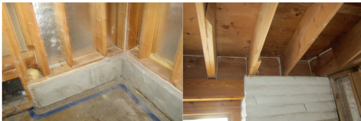
Seams are recaulked at sill and rafter ends.
