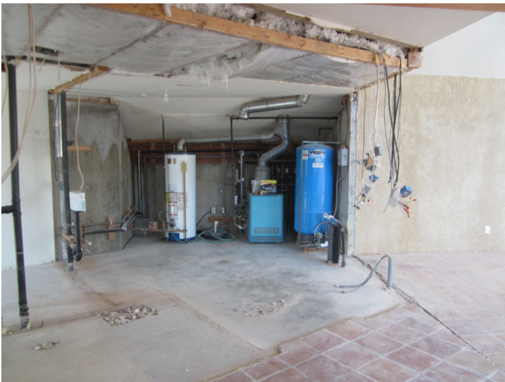
Example of attic blown in insulation over 2 x 4 rafters and 4 mil plastic—this attic was removed but there is another one over the crawlspace area rear bedroom and bath constructed the same way.
