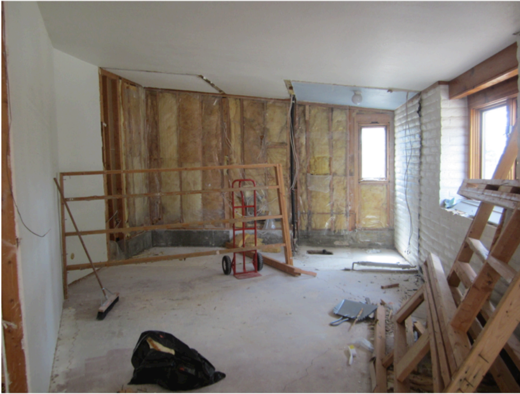
Existing unfaced fiberglass batt insulation installation in 2 x 6 studs, covered with 4 mil plastic.
