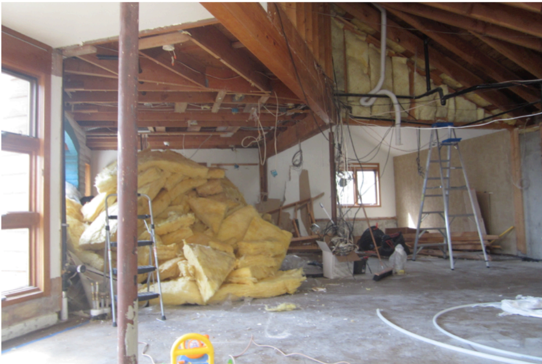
Fiberglass batts and plastic removed from slab area ceilings. The best batts were saved to provide more insulation for the remaining attic area and other outbuildings.
