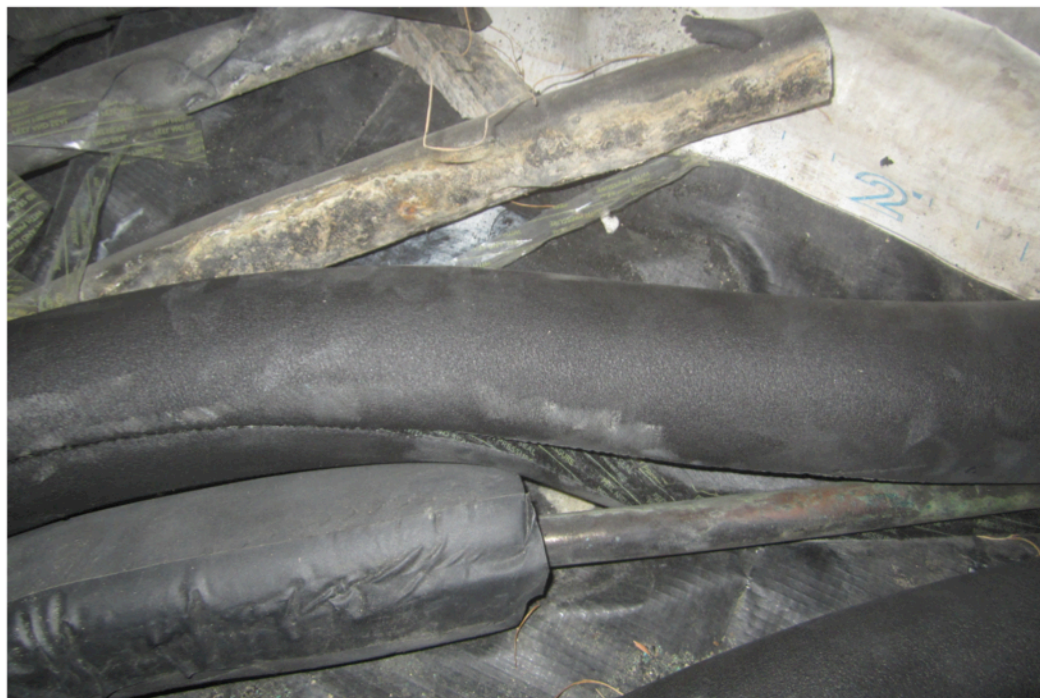
Old pipe insulation replaced with new R-7 pipe insulation.
