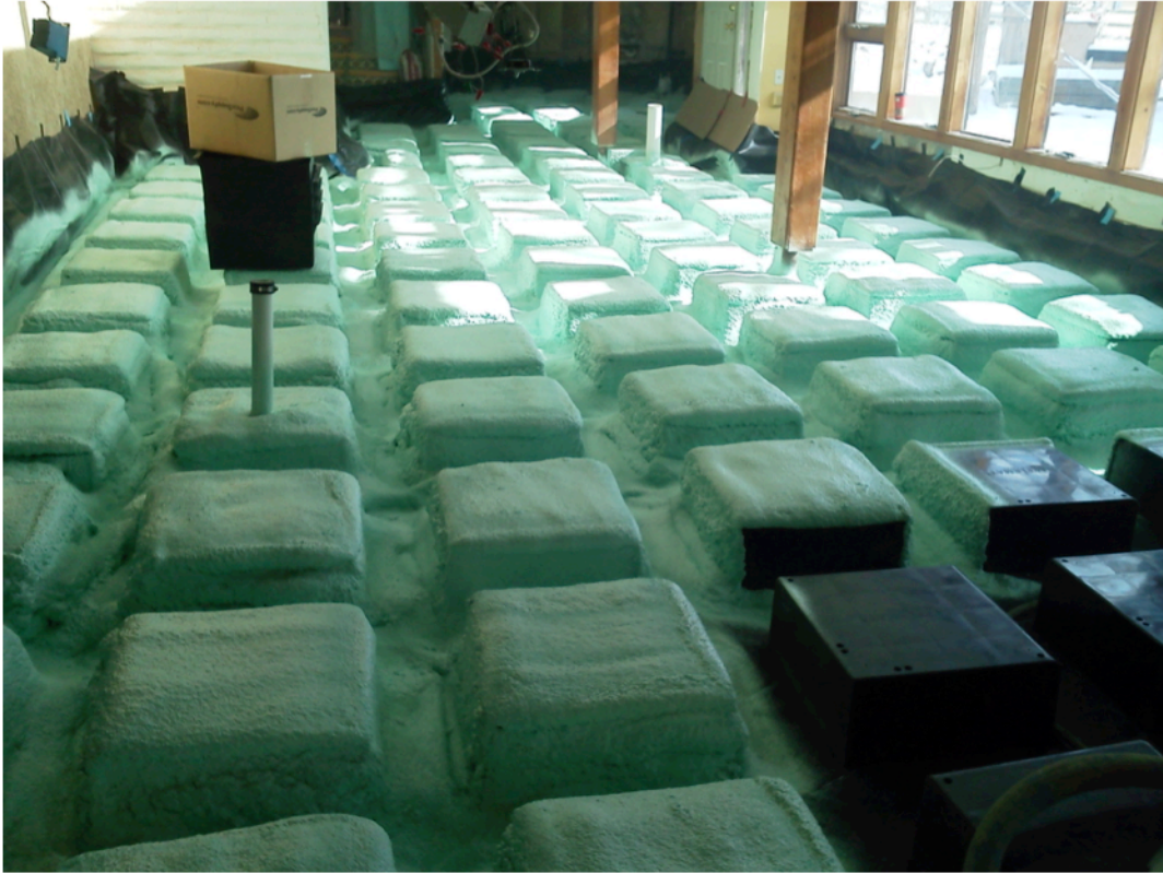
Two inches of closed cell foam was sprayed over the boxes and vapor barrier.
