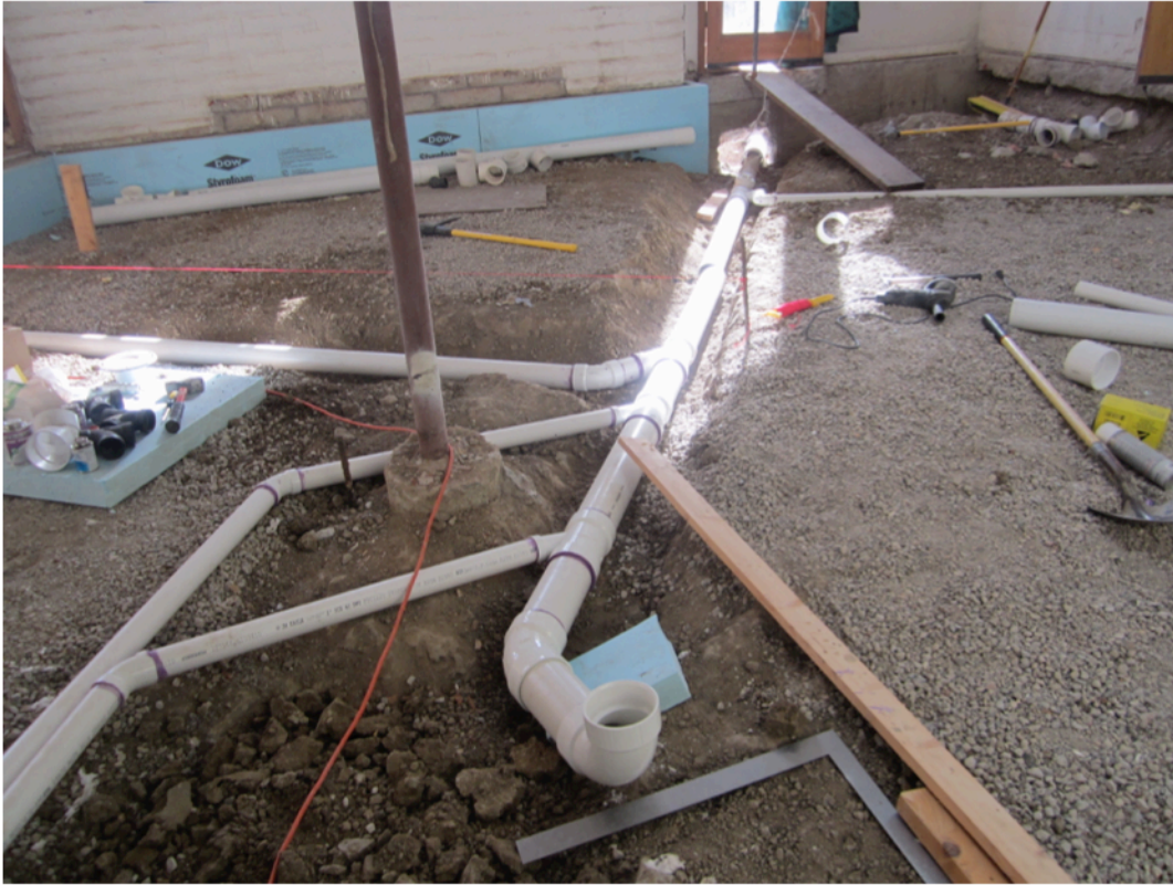
Recycled 3" XPS insulation was installed around the perimeter of the foundation.
