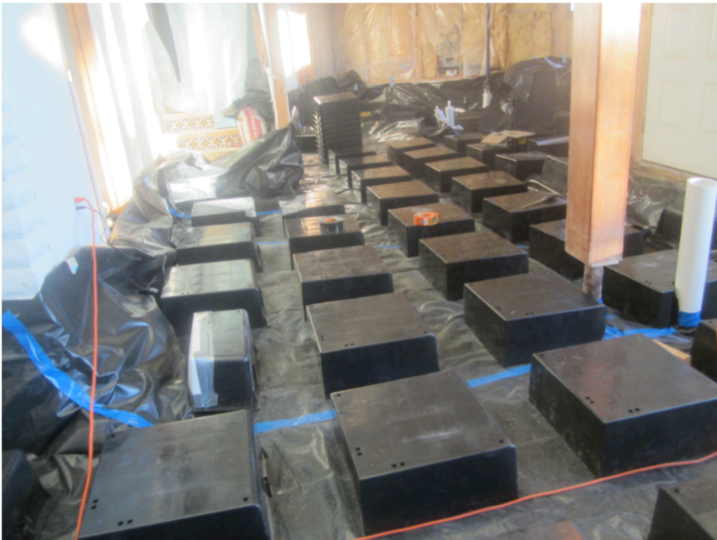
Recycled plastic Wafflemat boxes were installed over a machine tamped gravel bed and a 10 mil plastic vapor barrier that was overlapped and taped at the seams and around all plumbing penetrations.
