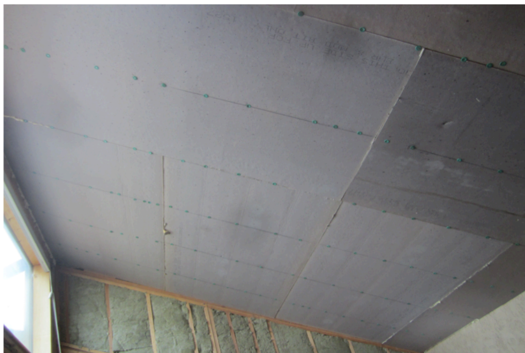
Recycled 1.5" (about R-9) polyiso installed on ceilings.
