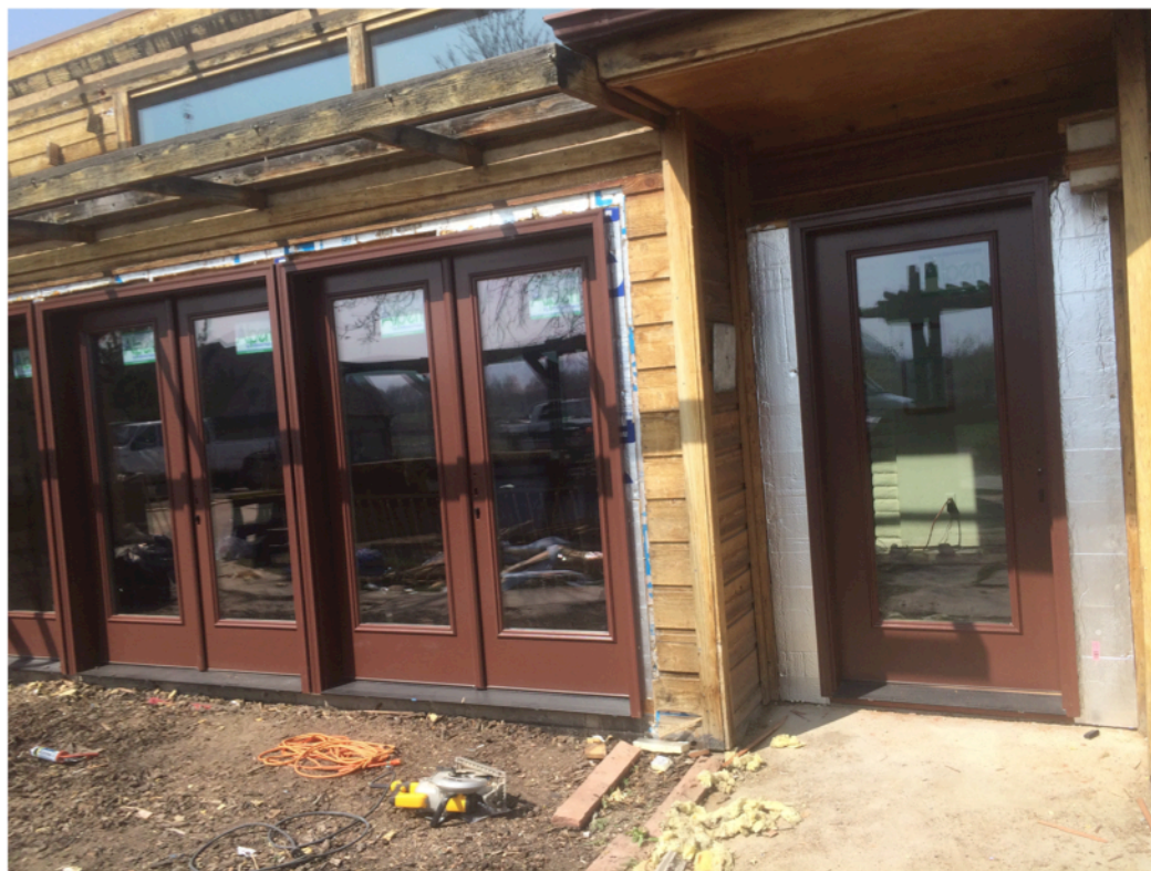
Ultra high efficiency Alpen windows and doors with SIGA tape and low VOC closed cell foam sealant.
