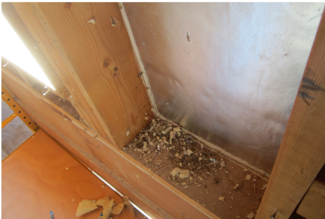
One inch polyiso sheathing on exterior is caulked at seams.
