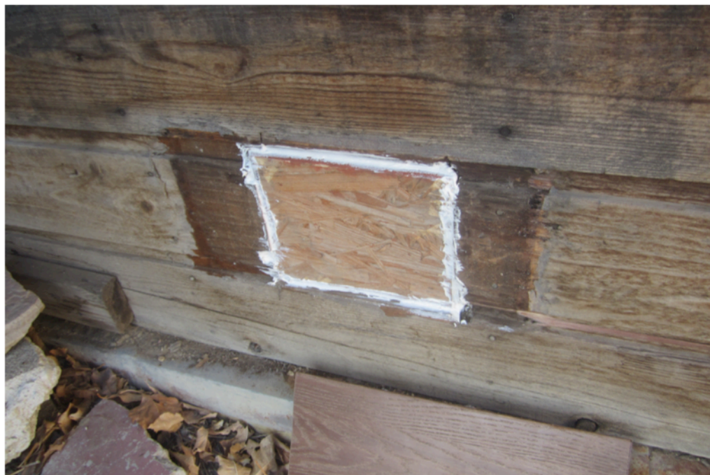
Crawlspace vent sealed.
