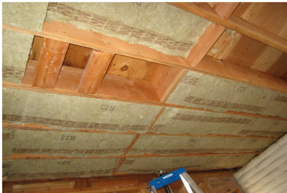
New Roxul rock wool insulation is installed in ceilings (R23) and walls (R-46).
