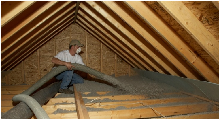
Cellulose, a fiber insulation material with a high recycled content, is blown into a home attic. | Photo courtesy of Cellulose Insulation Manufacturers Association.
