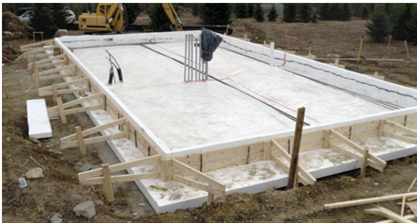
Figure 3. The author forms a monolithic, thickened-edge slab using 4-inch-thick foam board braced with framing lumber (top). After the air-vapor barrier is installed (above), the interior is filled with compacted gravel that's contoured to form the thickened edge. Long screws pushed through the vertical foam hold it to the hardened concrete.
