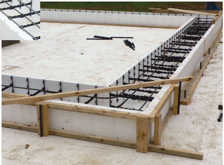
Figure 4. In this alternative to the monolithic slab method, ICFs outline the foundation and are poured first (left). Forms are stabilized with framing lumber cleats, staked through the foam into the gravel base. Corners require extra bracing (below). Like the footings, column pads are set directly on the foam (bottom). A foam wrap helps prevent the vapor barrier from tearing over rough edges (inset). On this job, an extra layer of 2-inch foam raises the nominal R-value by 10.
