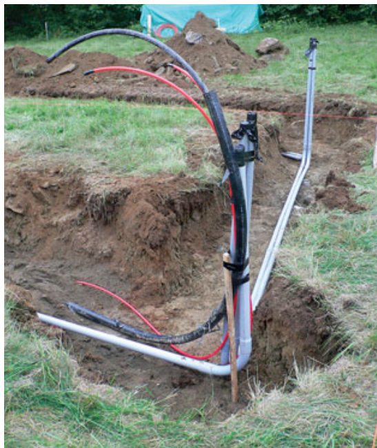
Figure 1. Water and utility lines are always placed first, eliminating later disturbance under the slab (above). On a relatively level lot, only minimal excavation is required (above right). The author occasionally uses a thin layer of flowable fill to create a void-free surface beneath the supporting foam layer (right).
