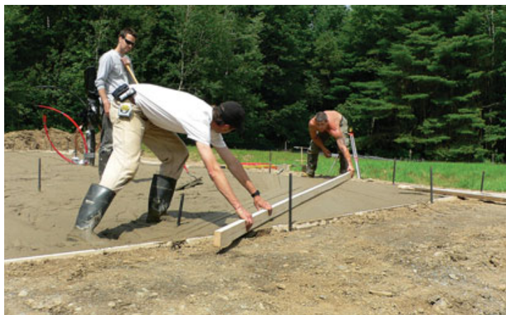
Figure 1. Water and utility lines are always placed first, eliminating later disturbance under the slab (above). On a relatively level lot, only minimal excavation is required (above right). The author occasionally uses a thin layer of flowable fill to create a void-free surface beneath the supporting foam layer (right).
