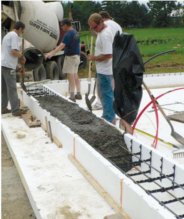
Figure 4. In this alternative to the monolithic slab method, ICFs outline the foundation and are poured first (left). Forms are stabilized with framing lumber cleats, staked through the foam into the gravel base. Corners require extra bracing (below). Like the footings, column pads are set directly on the foam (bottom). A foam wrap helps prevent the vapor barrier from tearing over rough edges (inset). On this job, an extra layer of 2-inch foam raises the nominal R-value by 10.
