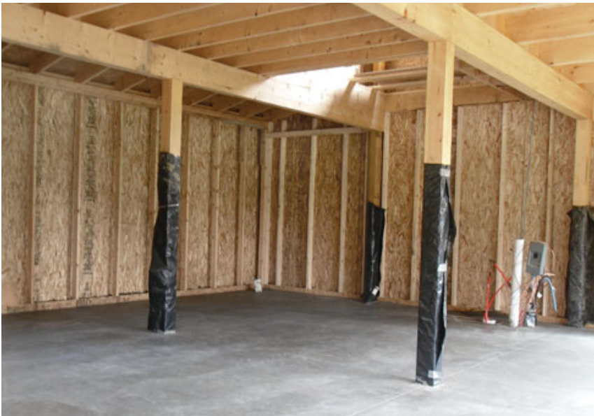
Figure 5. The ICF grade beam provides an immediate platform for framing (left). Once the building is enclosed, the slab can be poured without concern for temperature or foul weather (below).
