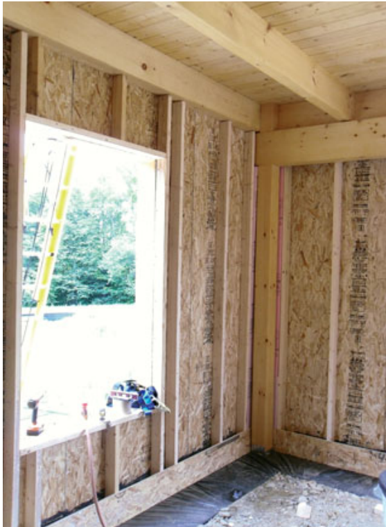
Figure 5. The ICF grade beam provides an immediate platform for framing (left). Once the building is enclosed, the slab can be poured without concern for temperature or foul weather (below).
