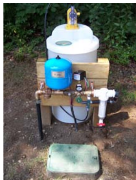
Iron stain prevention system installed outside near well/pump system (Tewksbury, MA)
