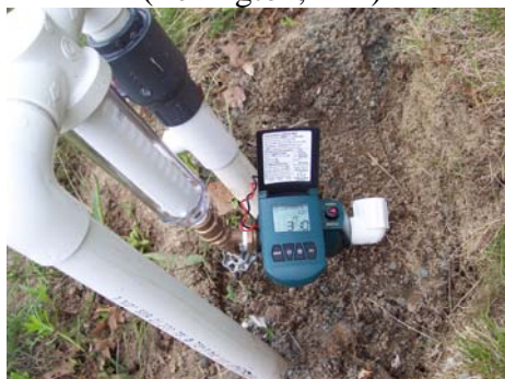
Automatic flush valve on sediment filter (Holliston, MA)
