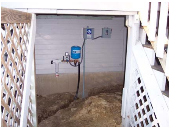
CPS including filter and electrical components mounted under deck (Sudbury, MA)
