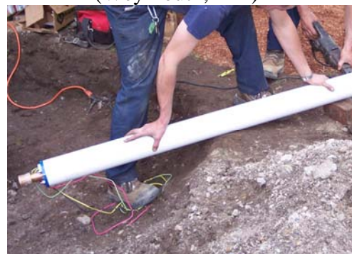
Screen being installed over submersible pump (Franklin, MA)
