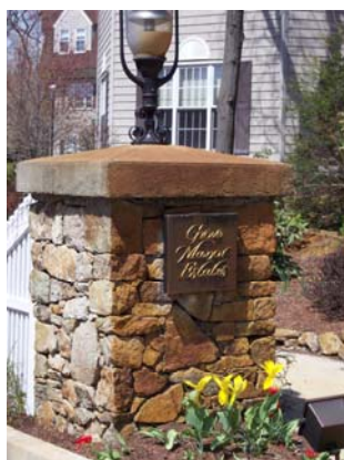
Iron staining on side exposed to irrigation system. Note the other side is not affected (Braintree, MA)
