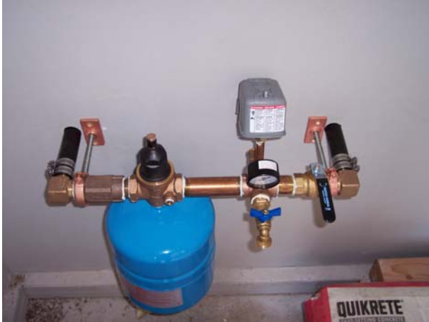
CPS mounted inside garage with sediment filter installed outside (Wayland, MA)
