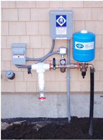
CPS on side of house with electrical components, disconnect and sediment filter (Milton, MA)
