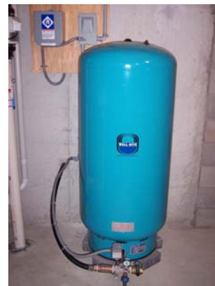
Large 119 Gallon Storage Tank installed in basement for home use (Mendon, MA)
