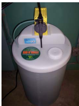
30 gal. tank with chemical feed pump and chemicals to eliminate staining, installed in basement (Lexington, MA)
