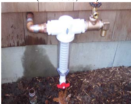
Sediment filter installed outside on side of house (Sudbury, MA)
