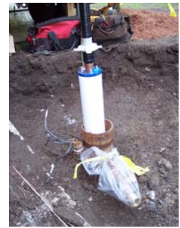
Drop pipe, wire guides, flow inducer, pump screen
