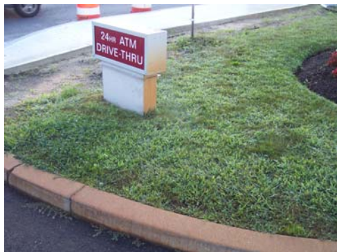
Iron stains to be removed from signage and curbing - notice sidewalk cleaned (Wilmington, MA)
