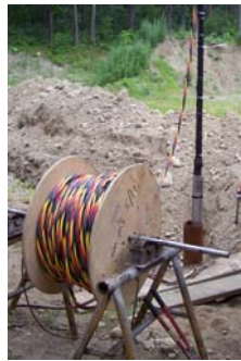
Drop cable, drop pipe and pump
