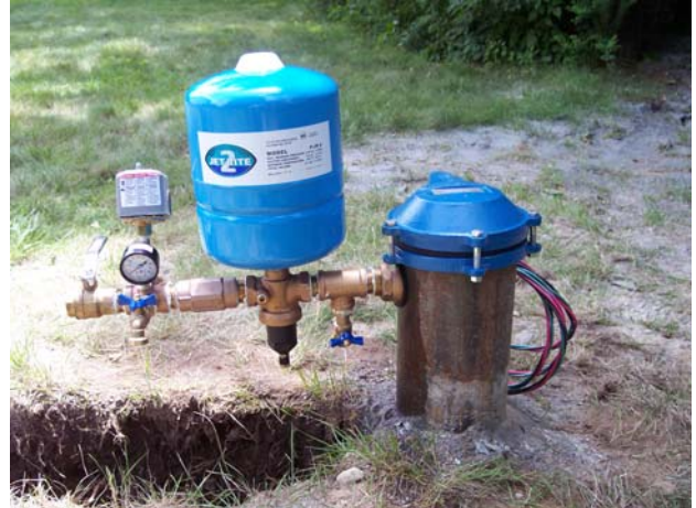
CPS mounted to well (Wilmington, MA)
