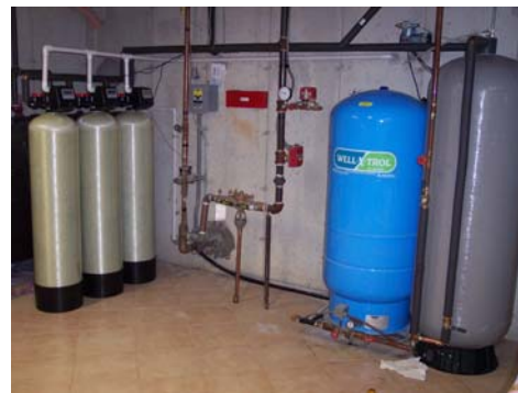
Iron removal system installed in basement of home (North Reading, MA)
