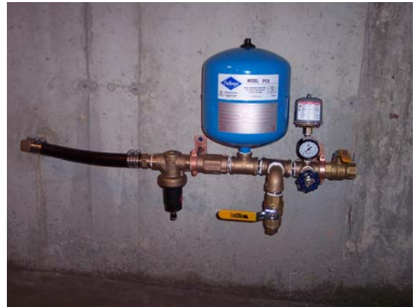
CPS mounted in basement of house with additional port for possible future expansion for home use (North Reading, MA)
