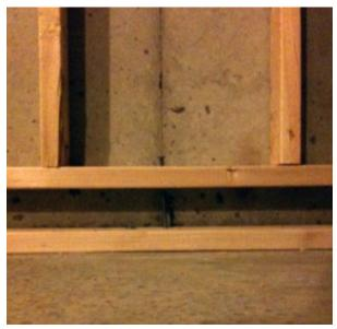
You now have a floating wall (you can also think of it as a hanging wall). As you will see, nothing is attached to the bottom base plate except the 60d nail. The nail will act as a guide rod should the concrete basement floor start to rise. However, it will not lift the top base plate because the 2×4 studs running to the ceiling are holding the top base plate in place.
