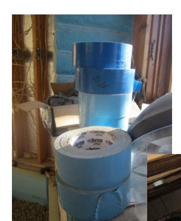
The crawlspace floor was covered with recycled billboard vinyl and taped with high quality plastic tape purchased from the Habitat Restore. This Bron tape is manufactured in Denver so it is also a local product. The light blue product is double sided. Some of the tape was yellow. I also used the tape to seal the vapor barrier that was placed over the compacted gravel under the new slab.
