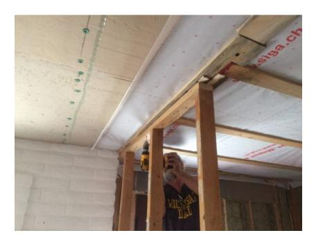
All of the studs from the existing walls in the house were saved and the nails were removed and recycled.
