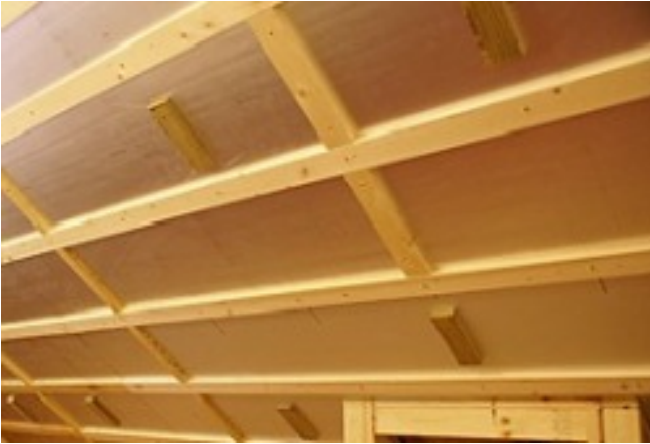
Polyiso retrofitted to a sloped ceiling
