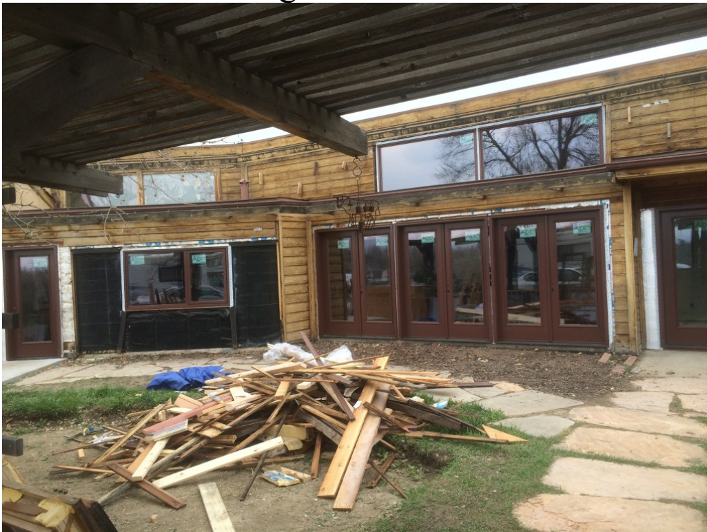
Windows and Doors at Installation
