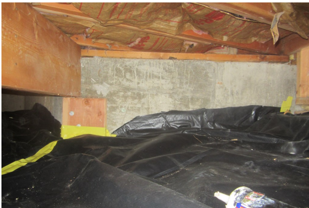
Vapor barrier caulked to walls
