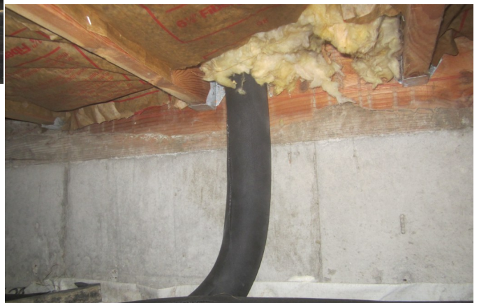
Thick R-7 insulation on water pipes
