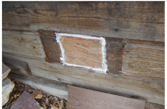
Outside vent removed
