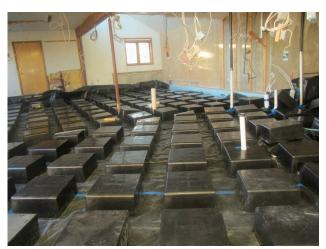
Recycled plastic boxes that are 19" x 19" X 8" tall are spaced 12" apart on a 10 mil vapor barrier over the plumbing and a rock layer and allow for soil expansion. After the old slab was removed an
