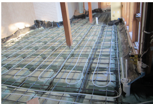
Radiant pipe design laid under concrete
