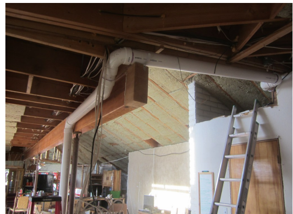
Radon vented to outdoor fan
