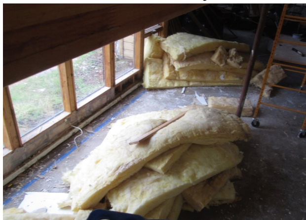
Reused fiberglass insulation
