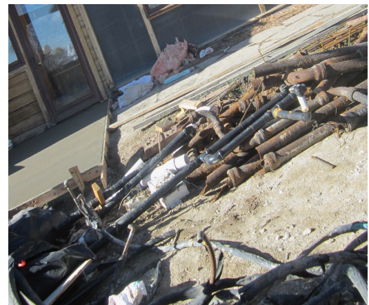
Recycled copper and metal
