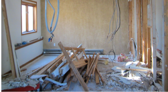
Reused 2x4's and trim
