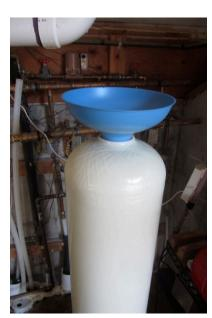
Our water is also above average in calcium carbonate and salts that the filter does not treat. A whole house carbon filter treats the water and the hot water side has a calcium filter. We use an electronic filter to keep calcium in suspension when it goes through our pipes. I learned that these work from the boiler manufacturer.
