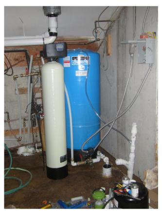
radon, but it does have a high concentration of magnesium and iron. To filter out these worst minerals the water filter is called MangOx from Clean Water Systems. The filter is filled with a greensand type of mixture that is chemically formulated to be more effective. A meter runs it every 600 gallons at 2 AM. It also has a chlorine rinse to help keep the
